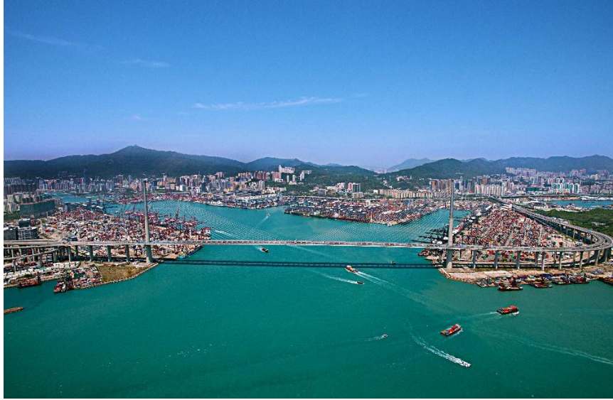
Aerial view of the Kwai Tsing Container Terminals
